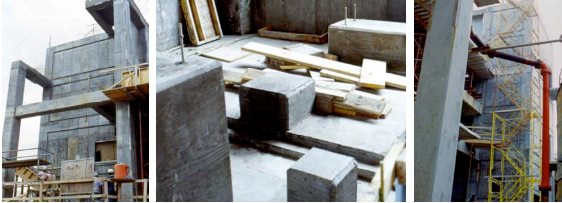
Fig 69-71 5-story chemical processing building entirely constructed with 22% silica fume HPC
