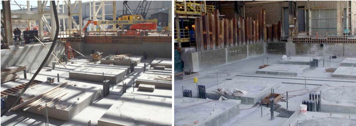
Fig 79-82 Titanium plant in Nevada undergoes retrofit with ultradurable high content silica fume concrete
