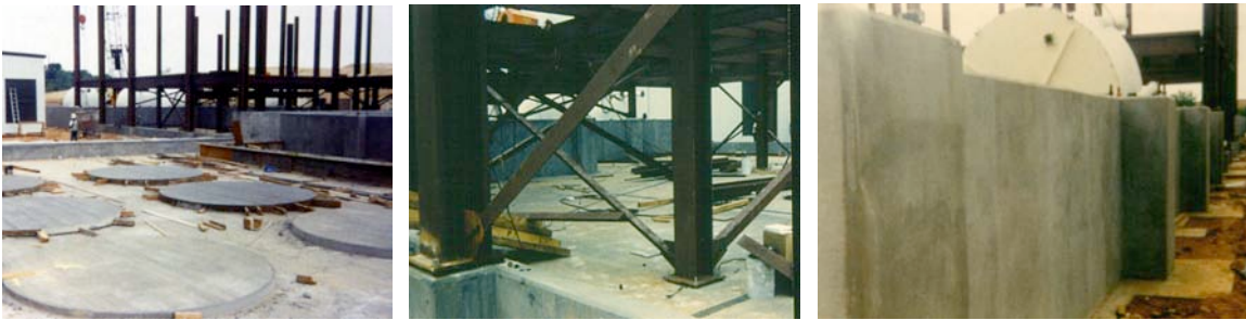
Fig 66-68 Chemical storage containment areas entirely constructed with a 10% silica fume concrete
