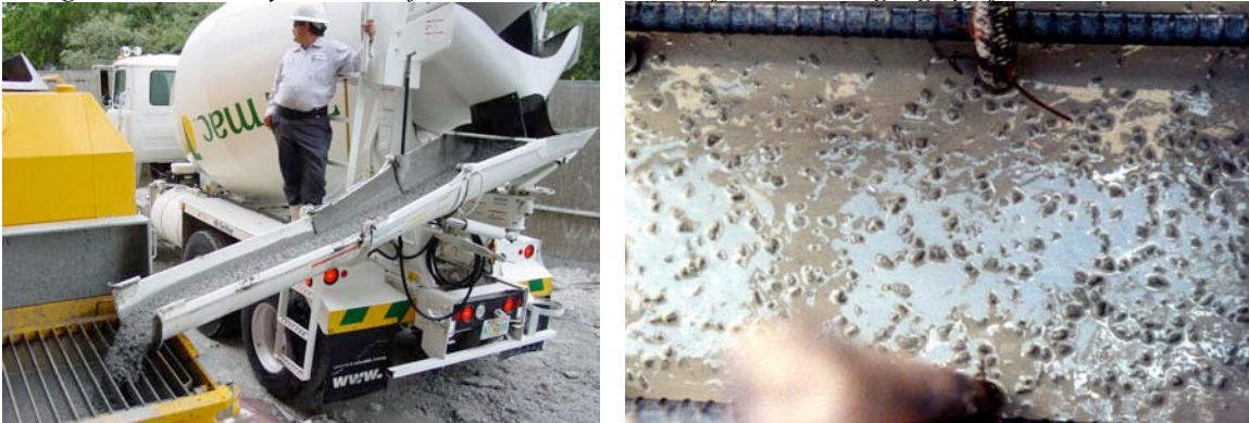
Fig 55-59 Extremely dense reinforcement necessitated self consolidating high performance concrete
