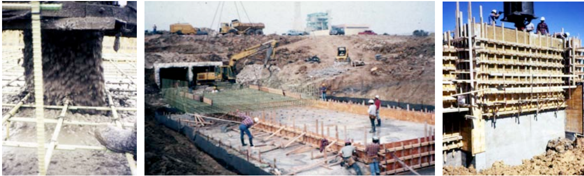
Fig.21-25 Texas' Calhoun County navigational district builds corrosion-resistant with silica fume concrete
