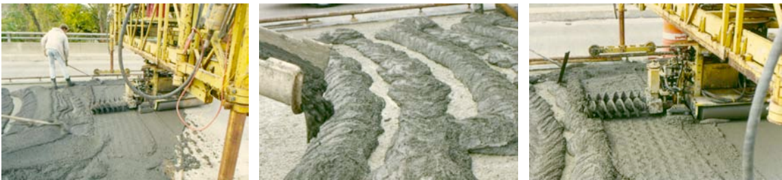
Fig.32-33 bridge deck machine takes over the leveling and screeding process; concrete deposits continue
