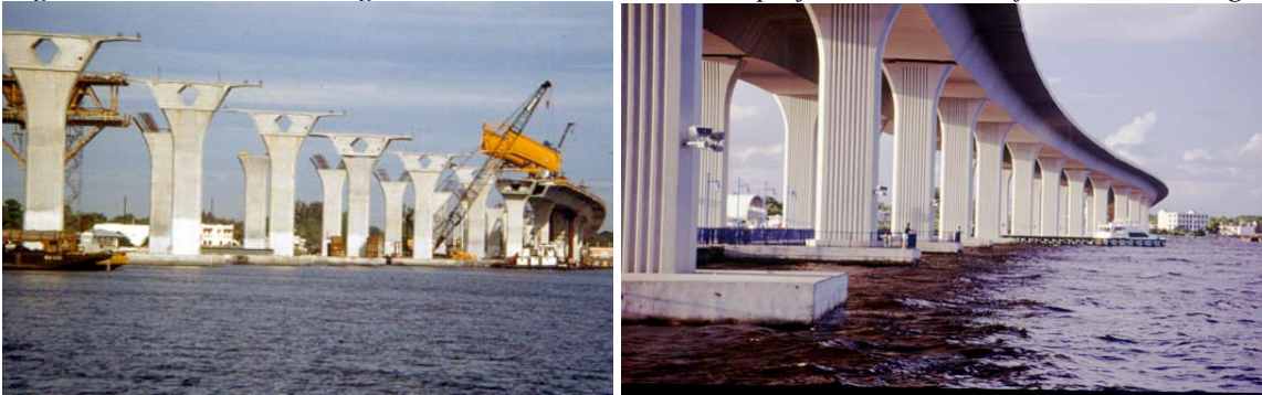
Fig.16-20 Mass concrete barged to location to Florida D.O.T. project at ocean inlet for new US 1 bridge
