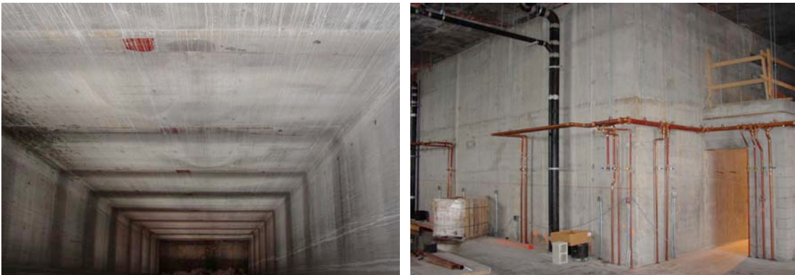
Fig 60-61 Cast-in-place silica fume SCC for elevator shaft (internal view) and 36th level transfer floor
