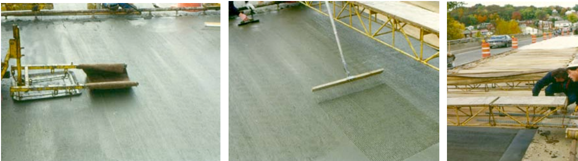
Fig.34-36 automatic float and burlap drag; final rake texturing; the critical curing via moist burlap cover
