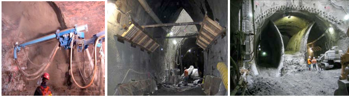
Fig.4-6 Robotic shotcrete application; inside and frontal view of sacrificial shotcrete walls support ATM
