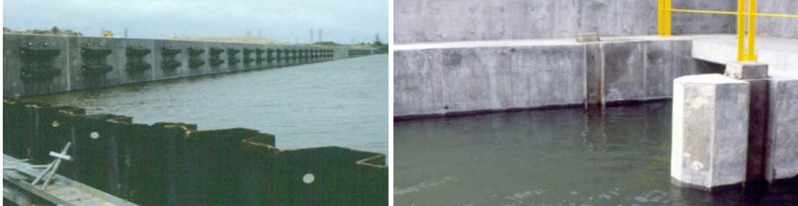
Fig.21-25 Texas' Calhoun County navigational district builds corrosion-resistant with silica fume concrete
