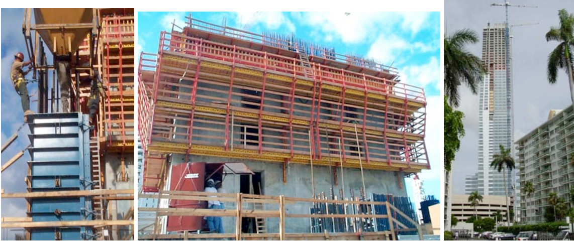
Fig 62-65 HPC column placement; external view of elevator shaft; nearly finished building in 2002
