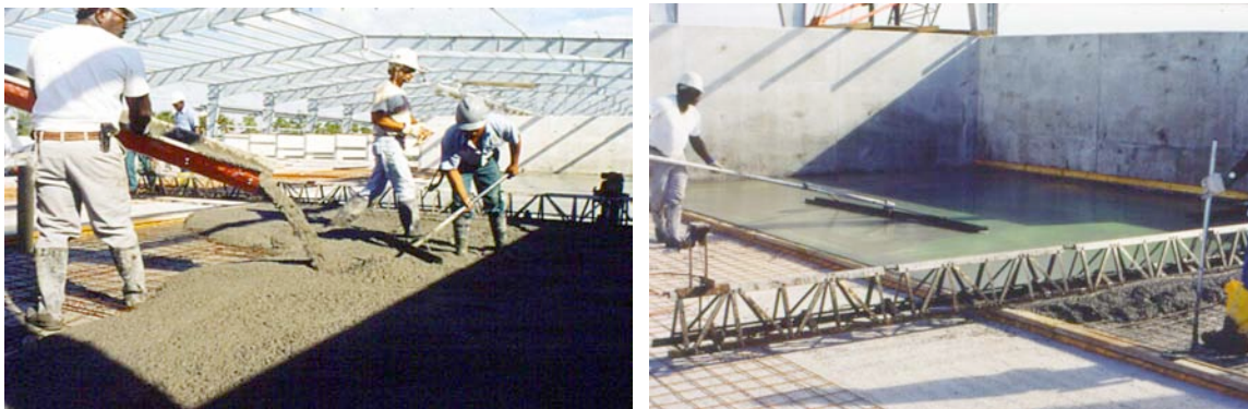
Fig 72-73 Compost transfer facility; pouring self-leveling concrete, followed by immediate final finish
