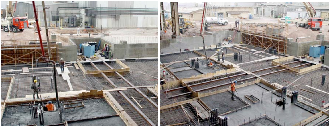
Fig 79-82 Titanium plant in Nevada undergoes retrofit with ultradurable high content silica fume concrete
