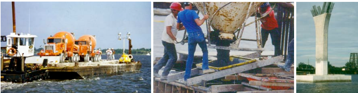
Fig.16-20 Mass concrete barged to location to Florida D.O.T. project at ocean inlet for new US 1 bridge
