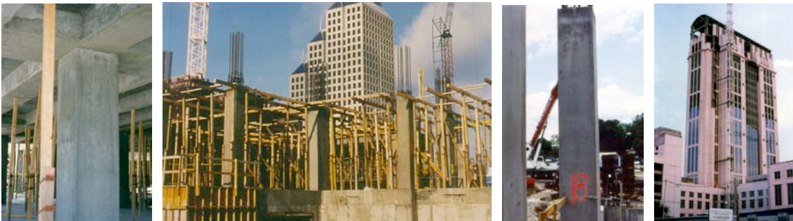
Fig 47-50 15,000 psi concrete for vertical applications at the Orange County Court House in Orlando
