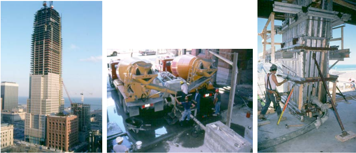
Fig 44-46 Society Tower; full height single stage concrete pumping and filling column from the bottom up
