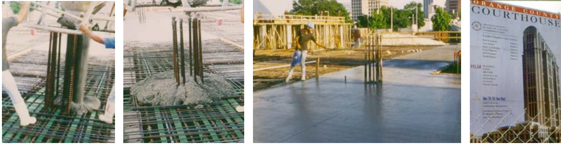
Fig 51-54 HPC concrete "puddling" for transfer of high strength concrete from columns through slab
