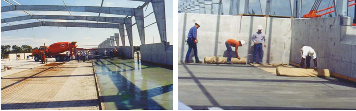
Fig 74-75 Two hours after bay 1 completion concrete can support manpower applying burlap for wet cure
