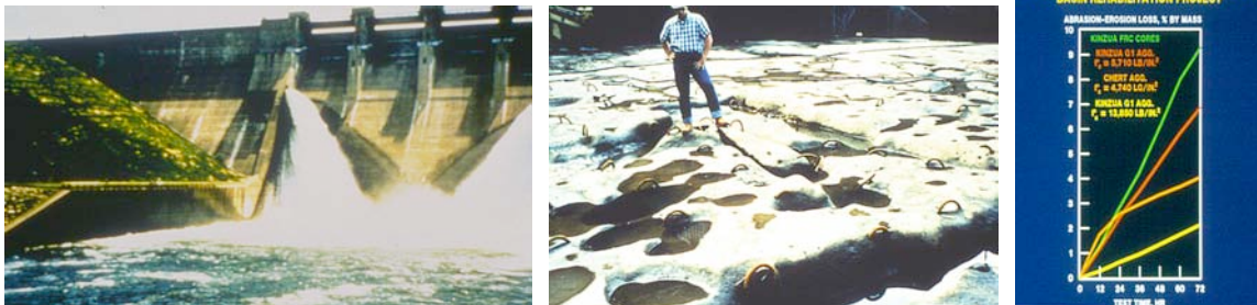
Fig.1-3 Kinzua Dam and de-watered stilling basin with severe erosion; Comparison of abrasion testing
