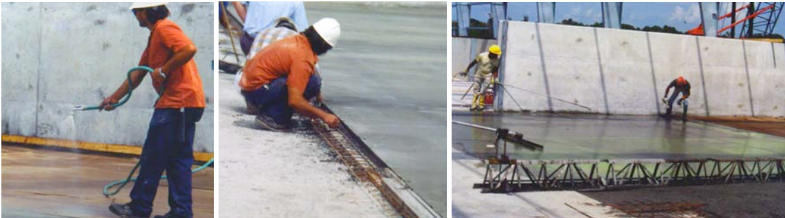
Fig 76-78 Two hours after bay 1 completion concrete can support manpower applying burlap for wet cure
