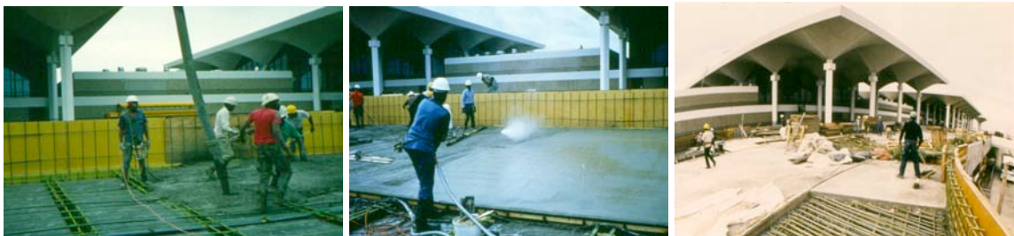
Fig.26-28 Memphis Airport; fogging concrete surface retains moisture, small sections to control cracking
