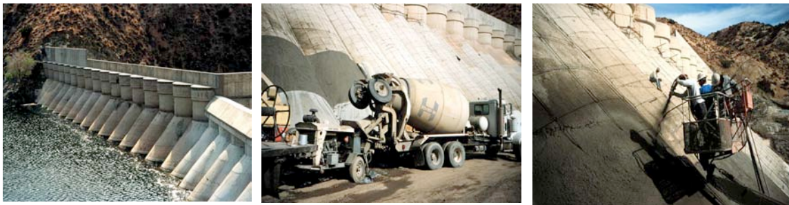
Fig.7-9 Little Rock Dam receives a seismic retrofit upgrade through ready-mixed delivered shotcrete
