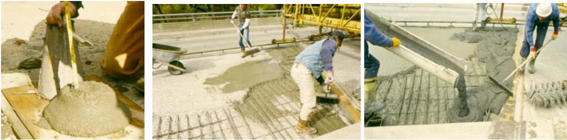
Fig.29-31 "medium" slump range \leq 8 "; bonding slurry application and concrete deposit close to location
