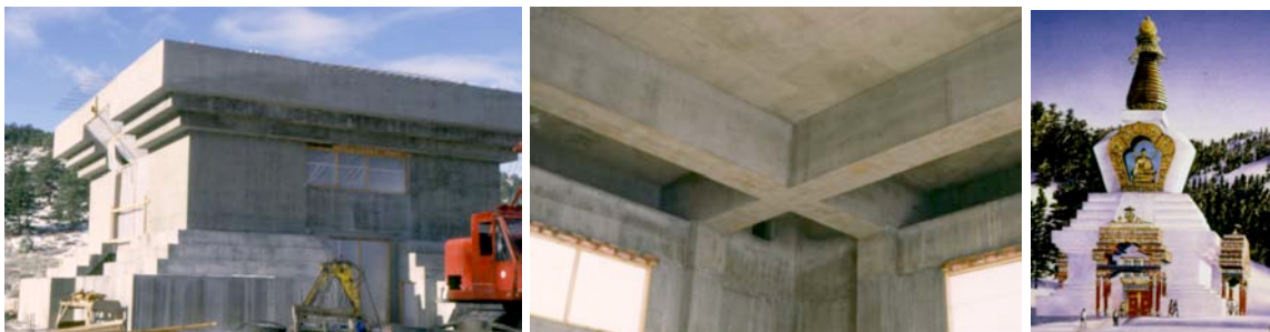
Fig.13-15 A 1000 year concrete design for the Great Stupa of Dharmakaya in Fort Collins, Colorado
